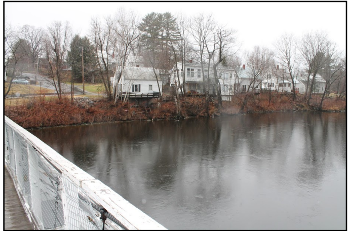
Steep shoreline on west bank of Kennebec River. Upstream shoreline anchor point for DV-01.
